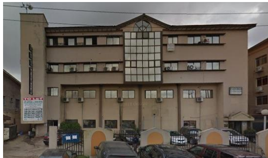
Figure 1: B&B Plaza (Building 1) Source: Field Survey (2022)
